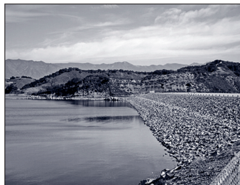
Picture of Casitas Dam showing lake level nearly full.
